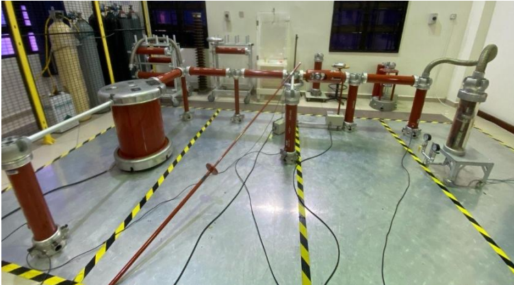
Figure 1.1: Single-stage circuit lightning impulse test setup of TERCO.
